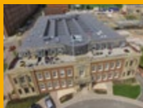
SINGLE PLY ROOFING
