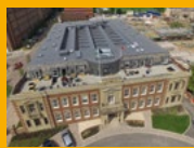
SINGLE PLY ROOFING
