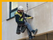
JOINT SEALING
