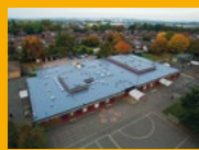
LIQUID APPLIED ROOFING
