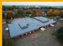
LIQUID APPLIED ROOFING
