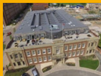
SINGLE PLY ROOFING
