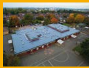
LIQUID APPLIED ROOFING
