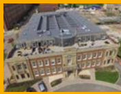
SINGLE PLY ROOFING
