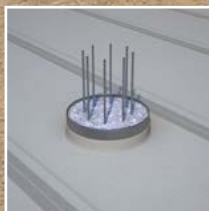
SikaProof® detailing solutions, e.g. for pile caps
